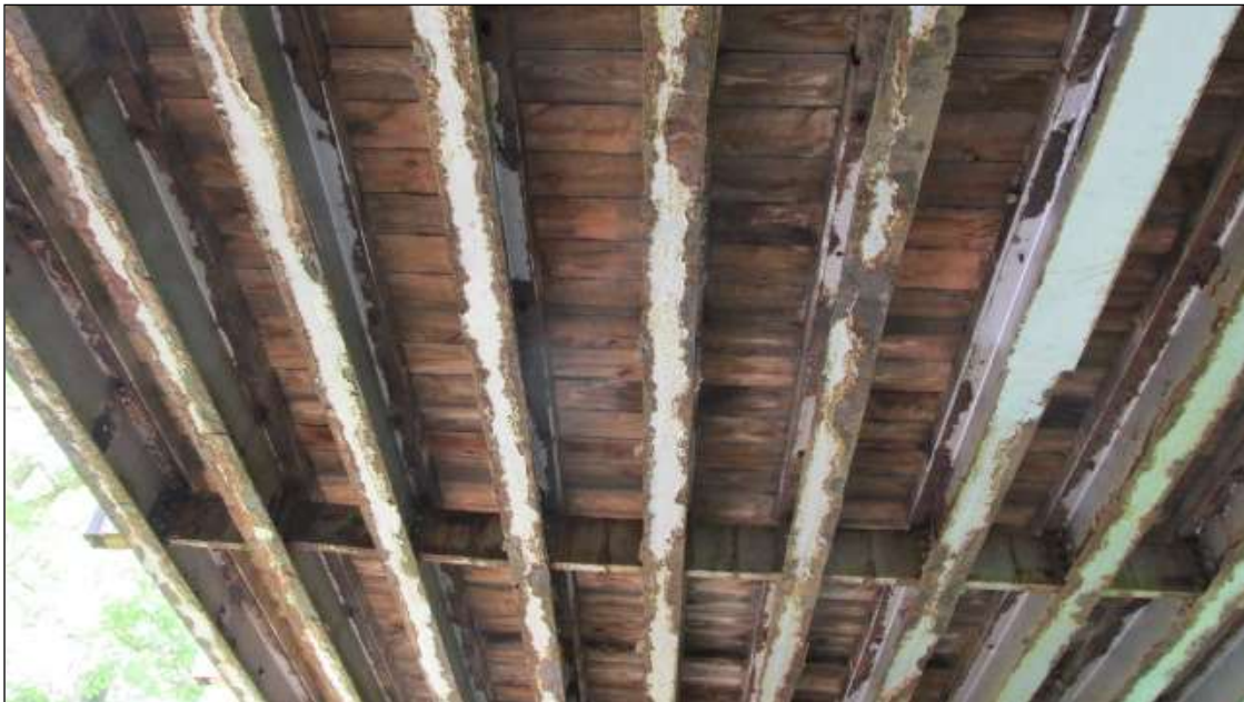
CORROSION ON BEAM FLANGES AND LOWER WEBS HAS FLANGES DOWN TO 3/16 INCH IN NUMEROUS AREAS
