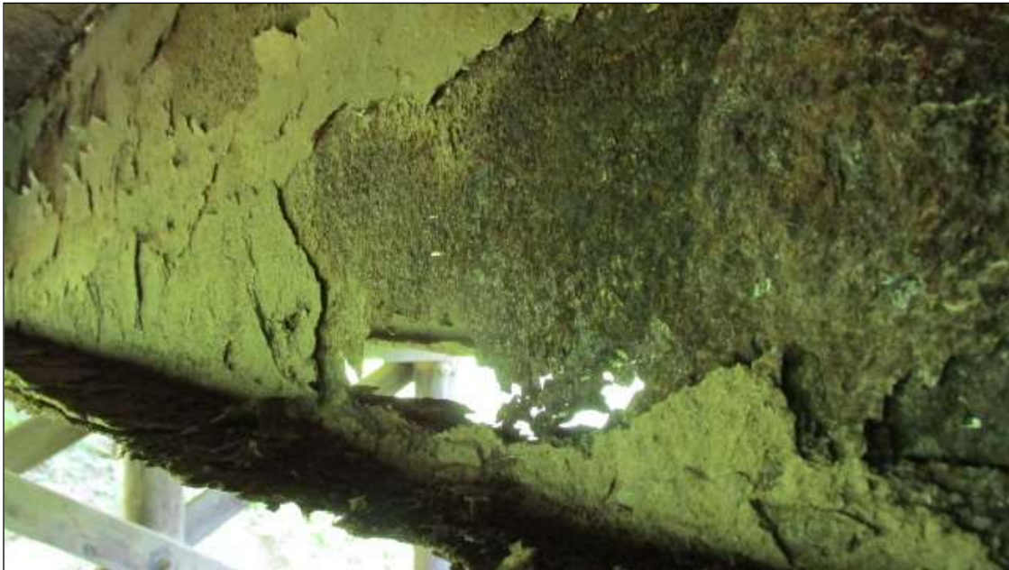
BEAM. 6 IN SPAN 3 HAS AREAS OF COMPLETE LOSS IN THE WEB. AT 12' FROM THE EAST END OF THE BEAM. THE LOSS IS 6" TO 8" LONG X 2" HIGH, NOTE THE WEB FACE
