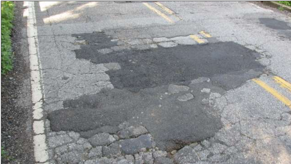
LARGE PATCHING AND ASPHALT WEARING SURFACE BREAKING OUT IN THE RT. LANE AT THE EAST END OF SPAN 3.
