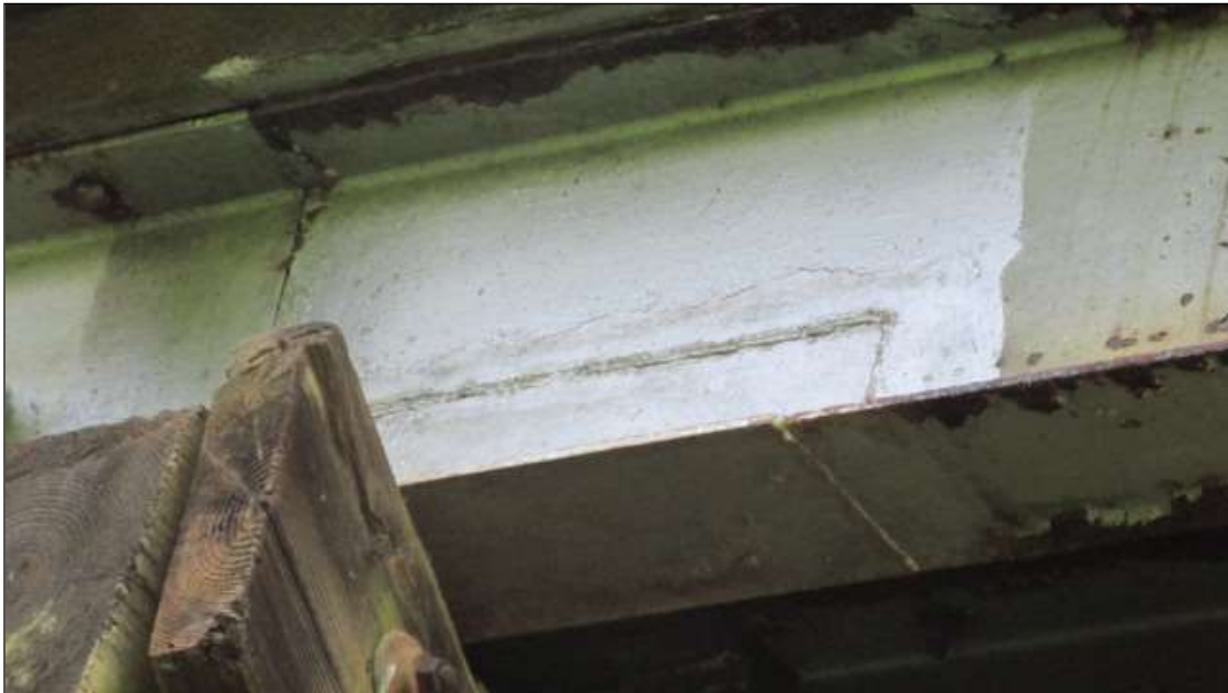
BEAM. 1 IN SPAN 2 AT BENT 2 HAS A PAST REPAIR WHERE THEY CUT AWAY DETERIORATED SECTION AND WELDED IN A SALVAGE SECTION. SALVAGE PIECE IS 6" HIGH X 18"
