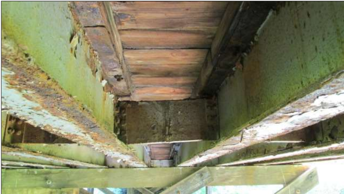
DIAPHS. HAVE SURFACE RUST AND PAINT. PEEL.
