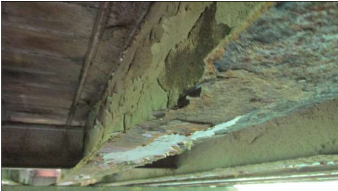
BEAM. 6 IN SPAN 3 HAS SECTION LOSS ALONG THE BOTTOM FLG. FOR 10" FROM 12' FROM THE EAST END OF THE BEAM., THE BEAM. FLGS HAS REDUCED DOWN TO A KNIFE ED
