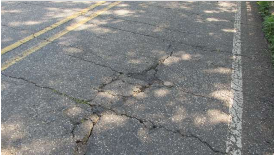
THE ASPHALT WEARING SURFACE IS BREAKING OUT IN ALL THREE SPANS, DECK IS REBOUNDING.
