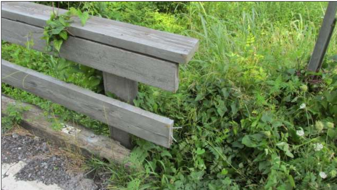
THE NORTHEAST PANEL BD. MISSING.
