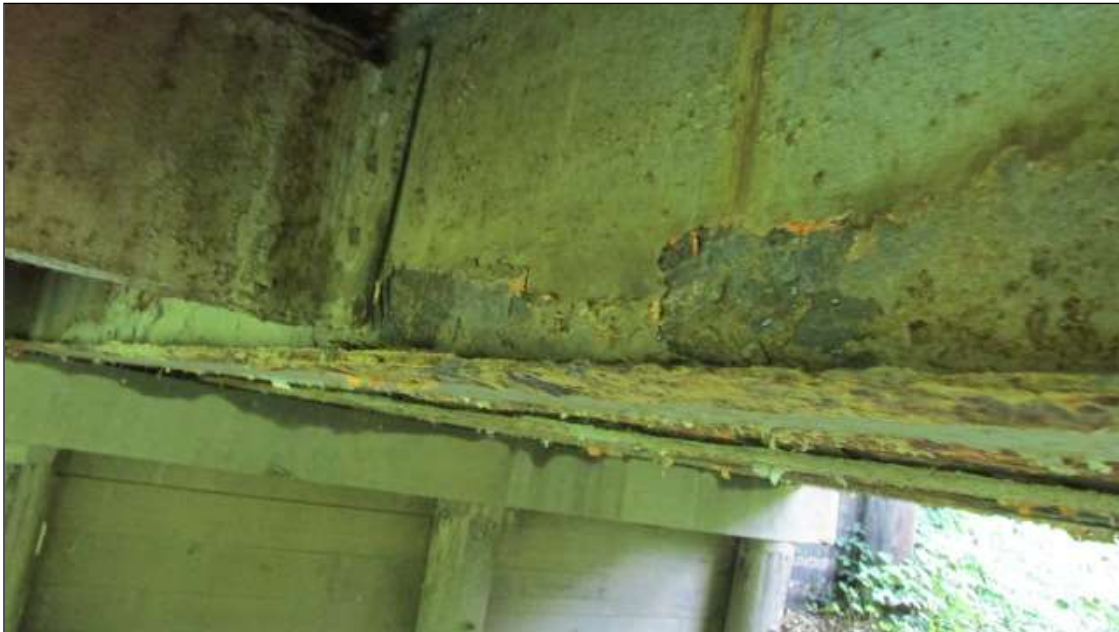
THE BMS. IN ALL THREE SPANS HAVE LAYERED RUST PRESENT ALONG THE TOP AND BOTTOM FLGS AND HAVE REDUCED DOWN TO A 1/8" FLG. THE WEB FACES HAVE SURFACE RU
