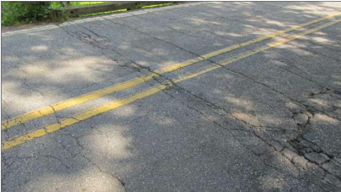
THE WEST APPROACH SETTLED ALONG THE FILLFACE.
