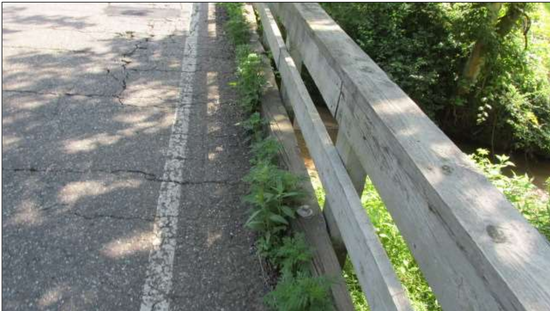
VEG. ALONG WHEELGUARDS HINDERING DRAINAGE.
